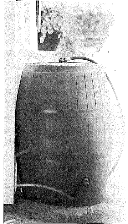
Figure 7-5. An example of a rain barrel receiving water from a downspout.
