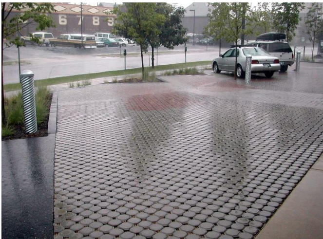
Permeable Pavement
